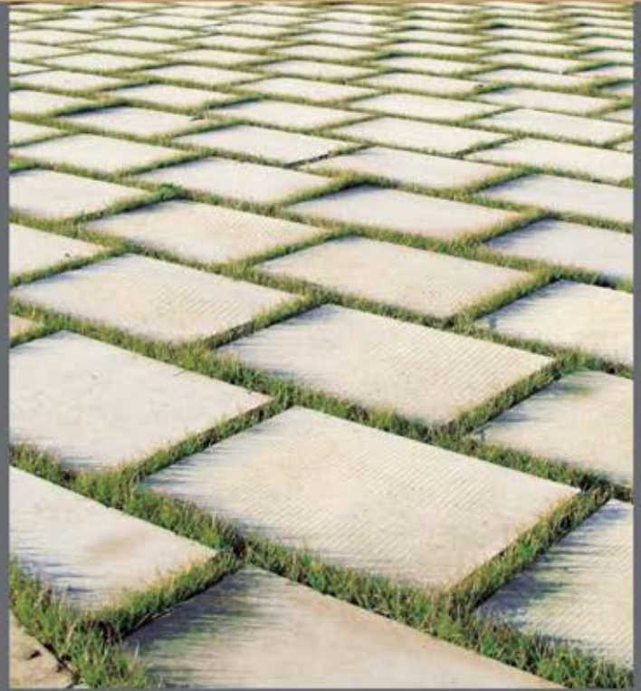
PAVIMENTO CALIBRATO CON FUGHE APERTE EXTERIOR FLOORING WITH SAW CUT FINISH 2 inches joint, with grass application.
